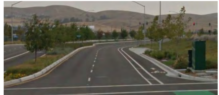
Example buffered bicycle lanes on Stoneridge Drive.
