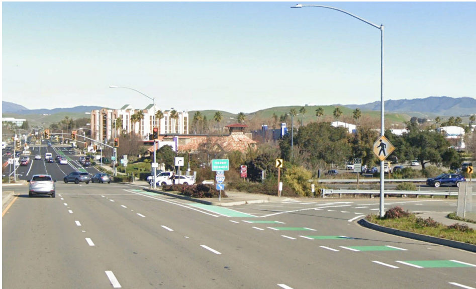
I-580 and Hacienda Drive Overpass
