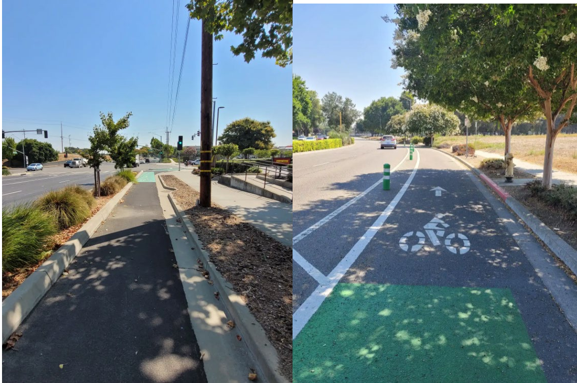
Street level bike lanes separated by curb (left) or flex posts (right)
