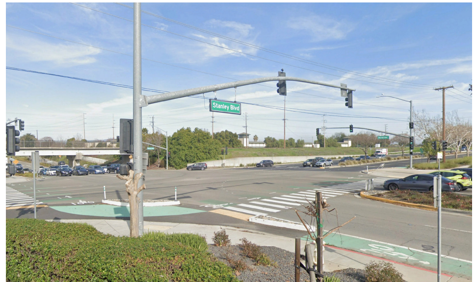
Intersection of Stanley Blvd and Valley Ave
