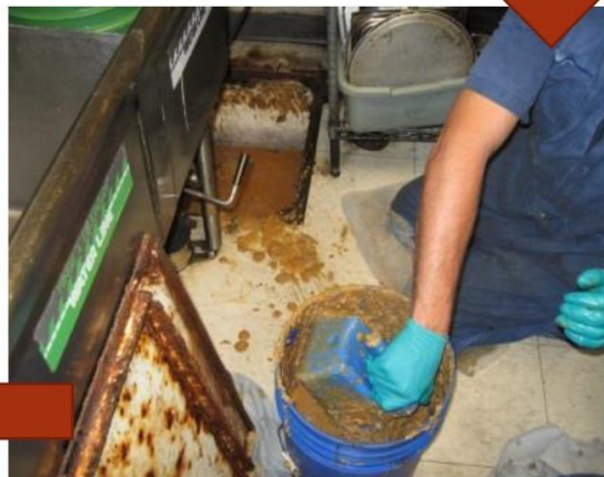
Remove solids from the bottom
