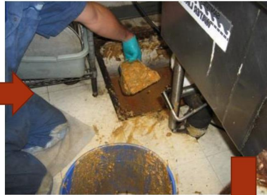
Remove grease from the top
