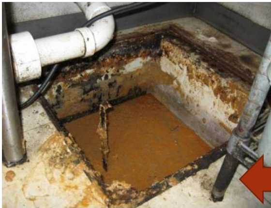
Scrape sides and inspect the interceptor
