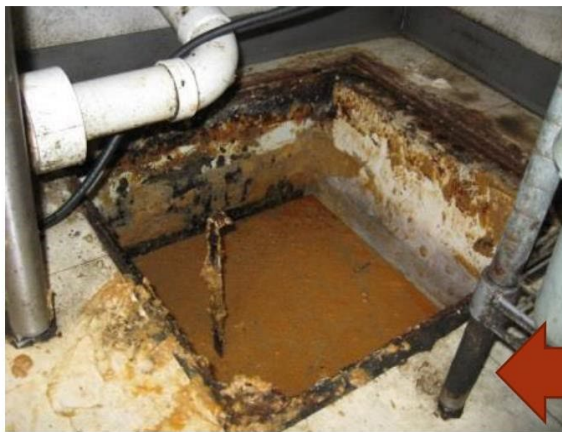
Scrape sides and inspect the interceptor
