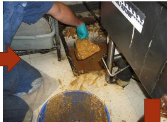
Remove grease from the top
