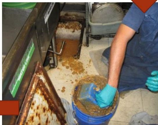
Remove solids from the bottom
