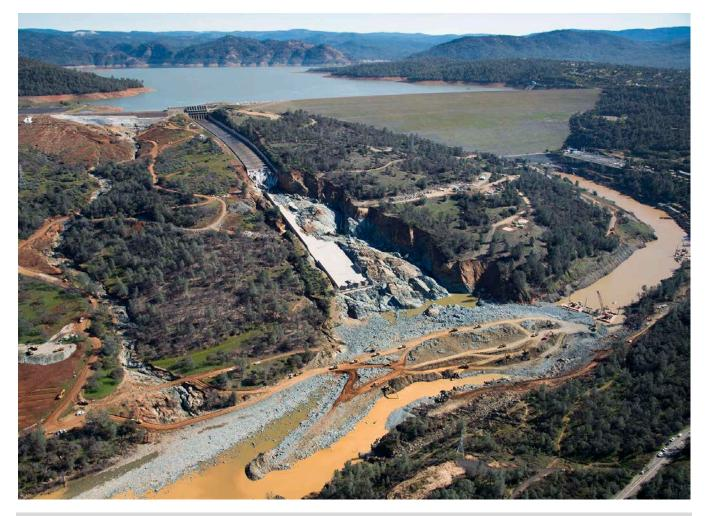
Figure 13-5. Oroville Dam Emergency Spillway Failure in Spring 2017
