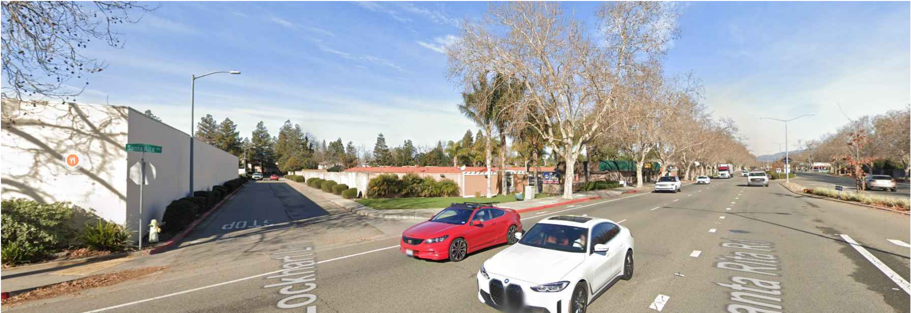
VIEW NO. 2 SITE LOCATION FROM INTERSECTION OF SANTA RITA AND LOCKHART LANE
