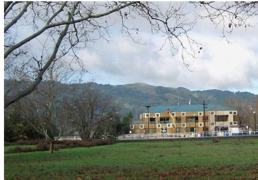
View of ridgeland behind Pleasanton Avenue commercial building
