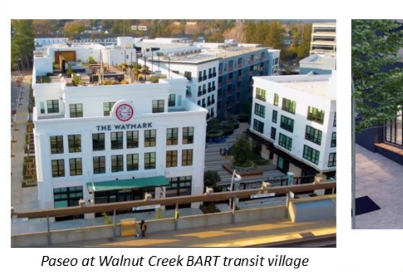
Paseo at Walnut Creek BART transit village
