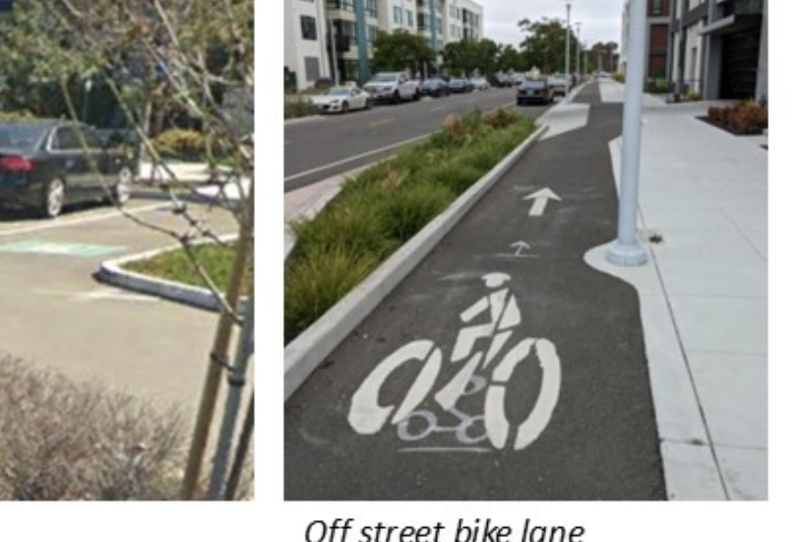
Off street bike lane
