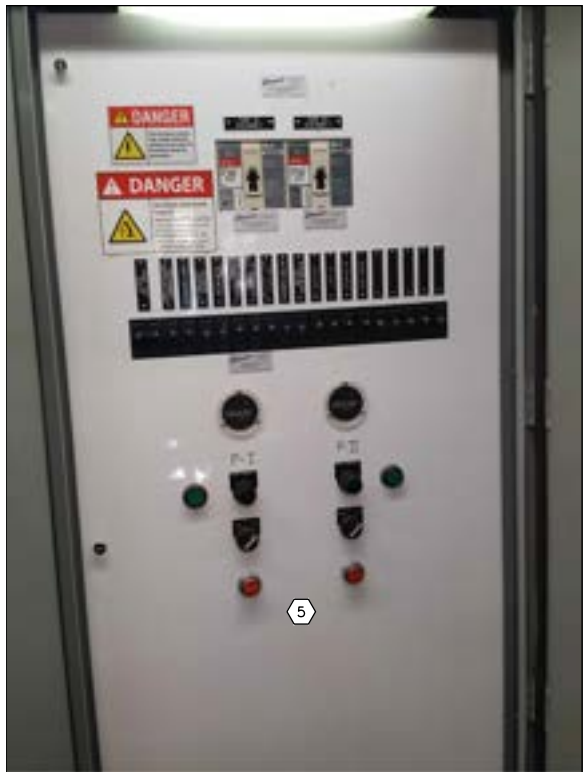
(G) S12 SEWER LIFT STATION (E) MOTOR CONTROLLER SCALE: NTS
