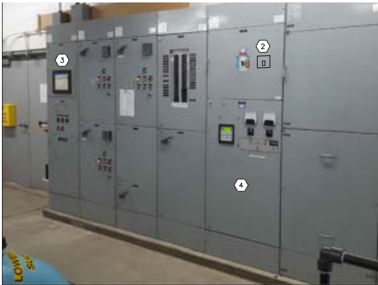
C LAUREL CREEK BOOSTER STATION (E) MOTOR CONTROL CENTER SCALE: NTS
