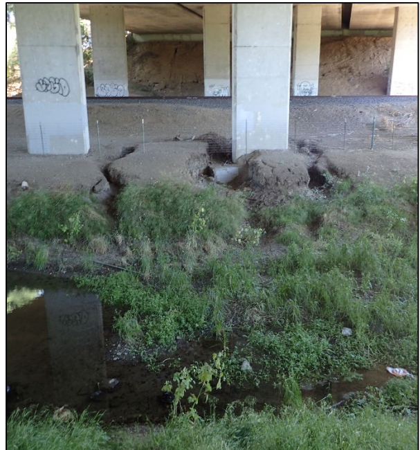
Photo 12: C-06 flowing under underpass
