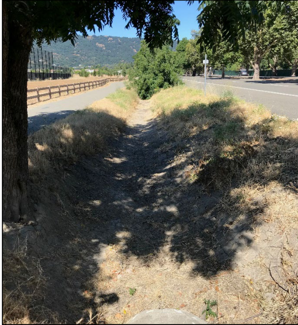
Photo 5: Excavated channel at Bernal V-Ditch (C-04)
