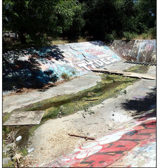
Photo 10: Manmade drainage at southern end of C-06
