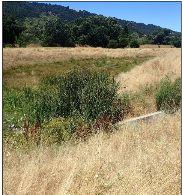
Photo 32: Culvert at P-04
