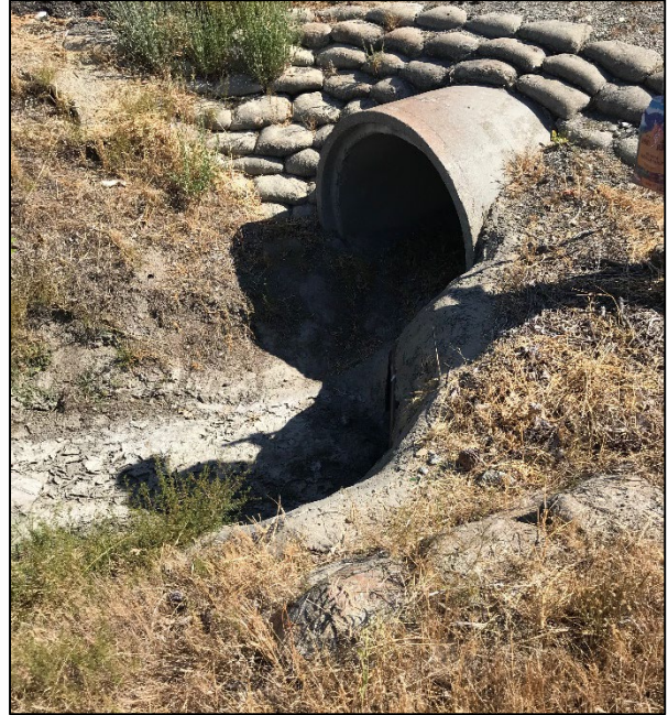
Photo 6: Culvert at C-04
