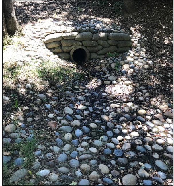
Photo 18: Bed and bank of C-09 lined with stones
