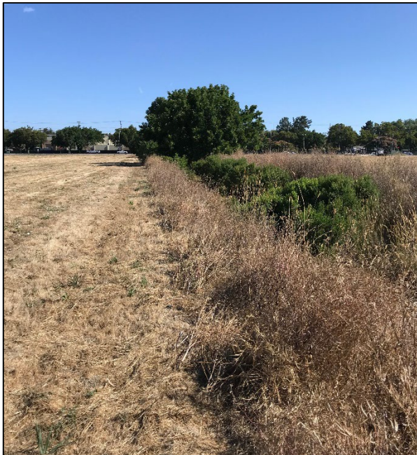
Photo 7: Excavated channel at Bernal North/South Ditch (C-05)
