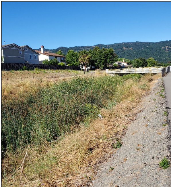
Photo 19: Junipero Canal (C-10)
