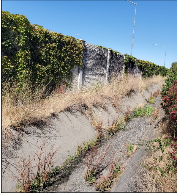
Photo 1: Concrete channel of Pimlico canal (C-01)
