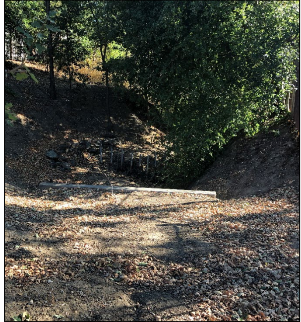
Photo 26: Rutledge Place Culvert (C-17)
