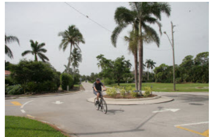
Example traffic circle, a traffic calming device that could be considered on a bicycle boulevard
