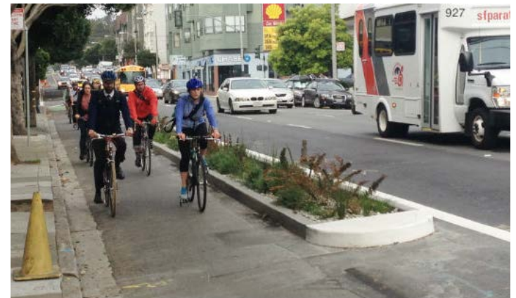
Bikeway separated by landscaping and raised concrete curb
