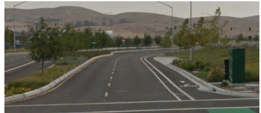
Example buffered bicycle lanes on Stoneridge Drive.
