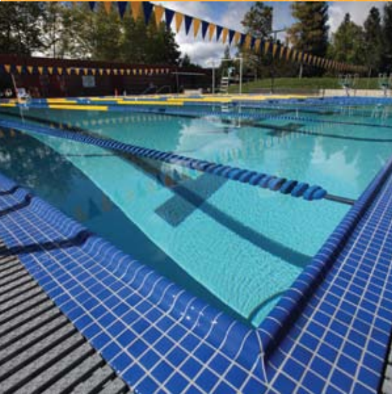
The newly renovated Dolores Bengtson Aquatic Center will serve the Pleasanton community for many years to come.
